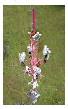
**Self-supporting towers** are legged pyramid-shaped lattice structures. This type of tower is commonly used to reach heights of up to 42 meters, although they can be built to reach greater heights. Self-supporting towers provide the most stability and are best suited for ground-level sites.
