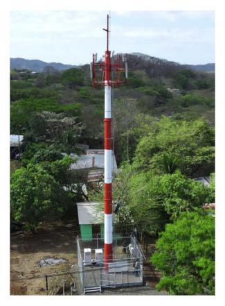
*Mastil towers* have a light composition, with a simple installation process and a very low cost. These types of towers are well suited for instances in which a high tower installation is not required (e.g., on rooftops). These towers are between 3 to 21 meters high and can be adapted to suit almost all project needs. It is important that this type of tower cannot support overly heavy accessories and other equipment.
