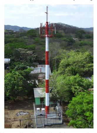
*Mastil towers* have a light composition, with a simple installation process and a very low cost. These types of towers are well suited for instances in which a high tower installation is not required (e.g., on rooftops). These towers are between 3 to 21 meters high and can be adapted to suit almost all project needs, although they cannot support overly heavy accessories and other equipment.
