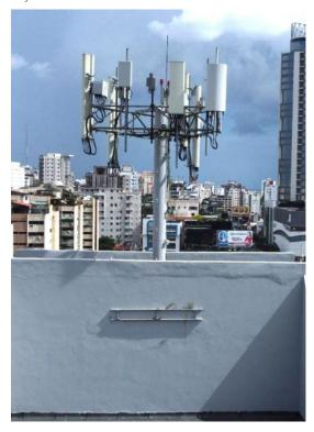
*Monopole towers* are conic-or constant-section round or polygonal tubular structures. This type of tower is commonly used to reach heights of up to 36 meters, but is only used where the amount of space a vailable is limited. It is the least-intrusive and easiest to assemble type of tower and is usually built on ground-level Sites.
